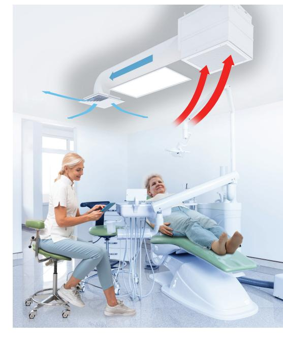
contaminated air is drawn away from the dental practicioner, and filtered air should be supplied from behind the patients head to wash the work space with clean air.
