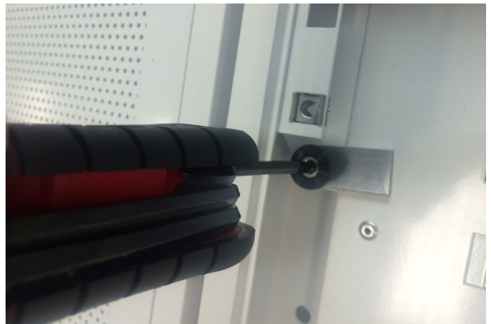
Replacement of Damper Assembly 2
