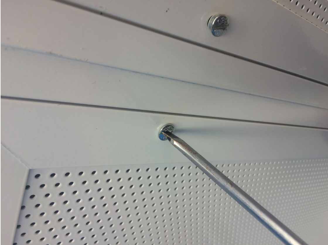
Fig. 3: Diffuser Face Removal
