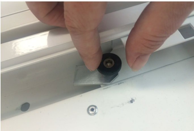
Replacement of Damper Assembly 1
