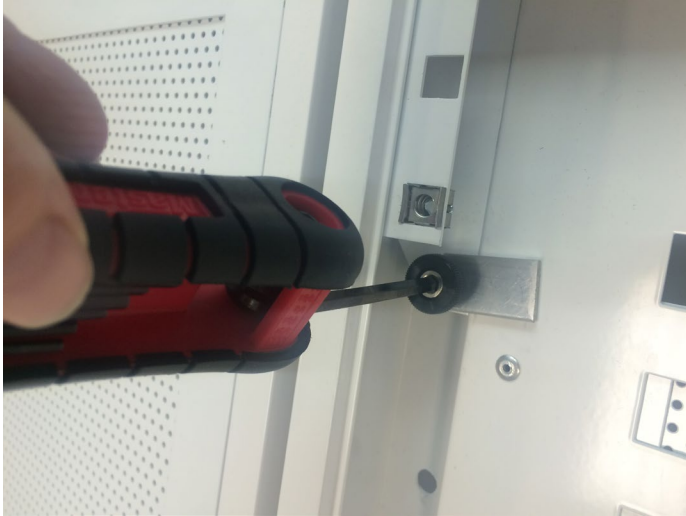
Loosen Knurled Thumb Screw
