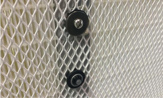
THREADED STANDOFF THROUGH FILTER CHANNEL ▼
