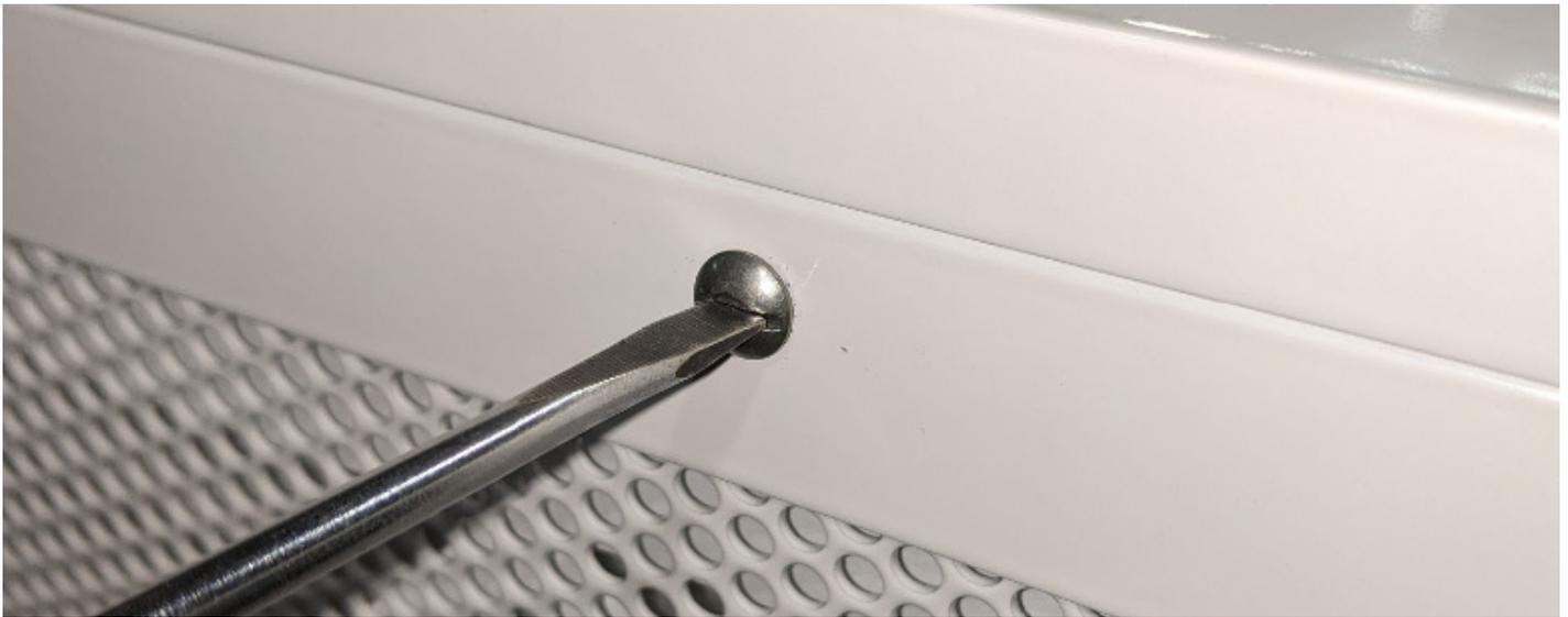
**Step 2:** Remove filter by loosening cam latch bolts (filter retainer clips) by turning counter clockwise using your hands, or hex key as required to fully tighten latches.
