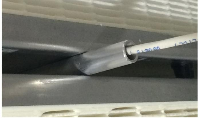
**Step 6:** With two (2) people holding the unit, pull cable back through plenum until plenum can rest on top of filter.
