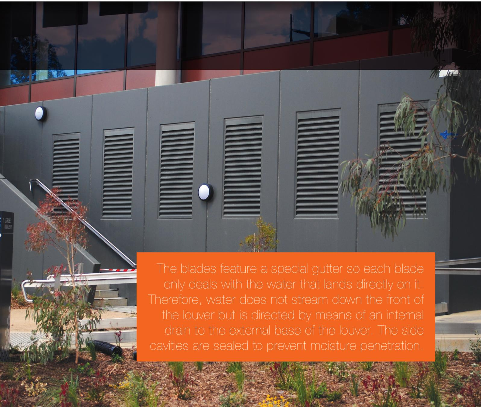
The blades feature a special gutter so each blade only deals with the water that lands directly on it. Therefore, water does not stream down the front of the louver but is directed by means of an internal drain to the external base of the louver. The side cavities are sealed to prevent moisture penetration.
